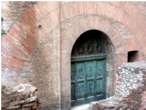
Relieving Arch over Doorway at Rear of Pantheon Showing Brickwork over Concrete Core. Wikimedia Commons. Anthony M. Cc-by-2.0
