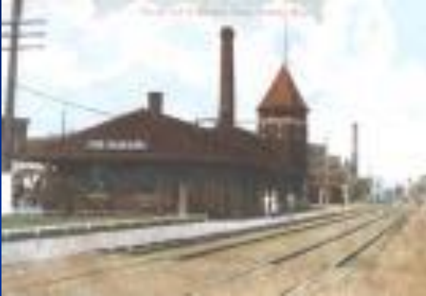
Old Chicago Rail Marshalling Yard
